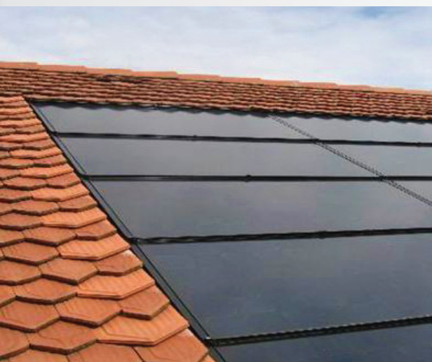
Sistema In-roof SL BIPV
